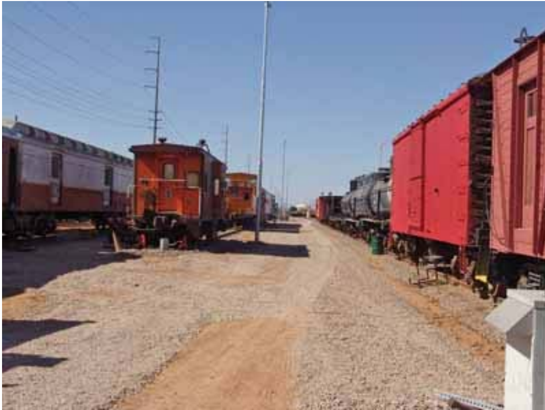
The grading between tracks 2, 3 & 4 are almost done.
