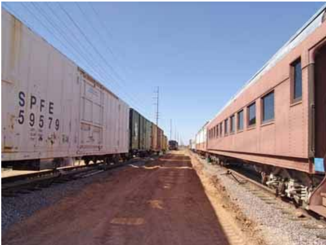
Dirt has been laid out waiting for gravel between tracks 1 & 2.
